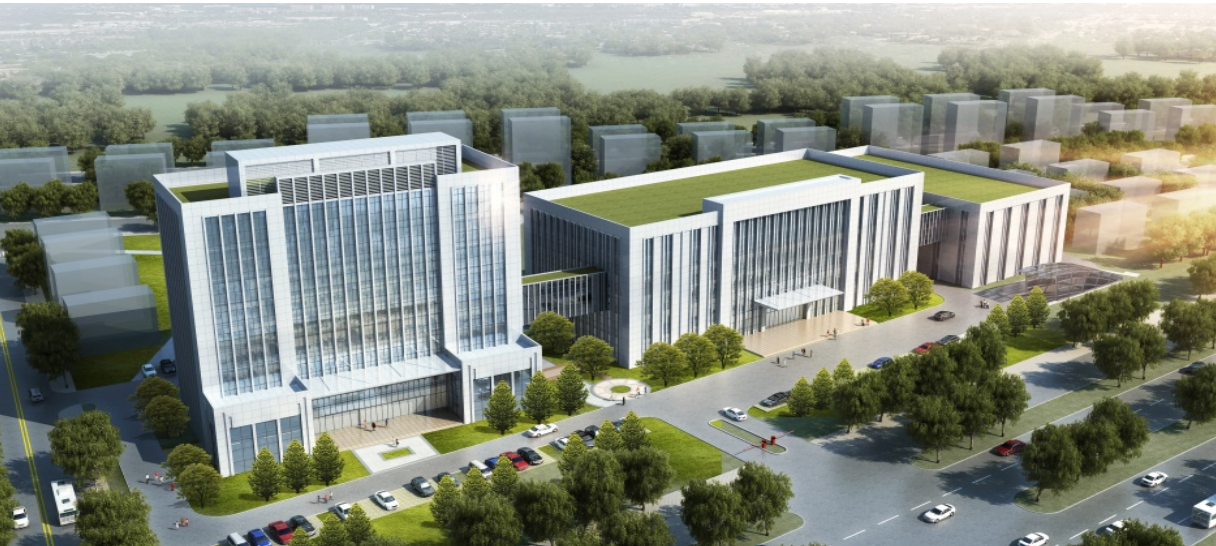
China Unicom Hengyang Big Data center
