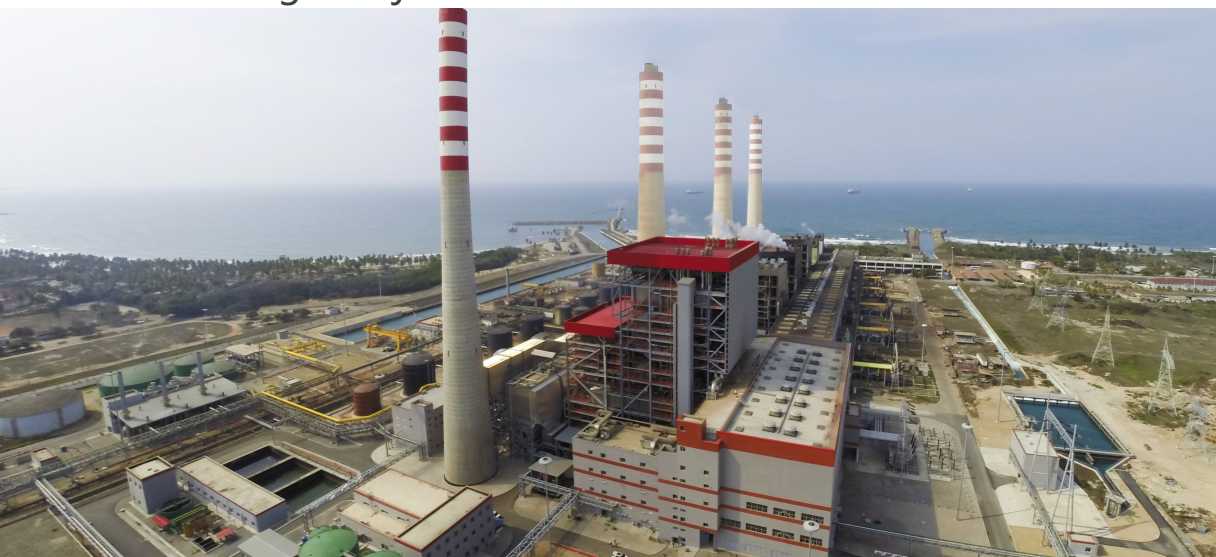
Project of 600MW Steam Turbine Power of Centro Power Plant, Venezuela
