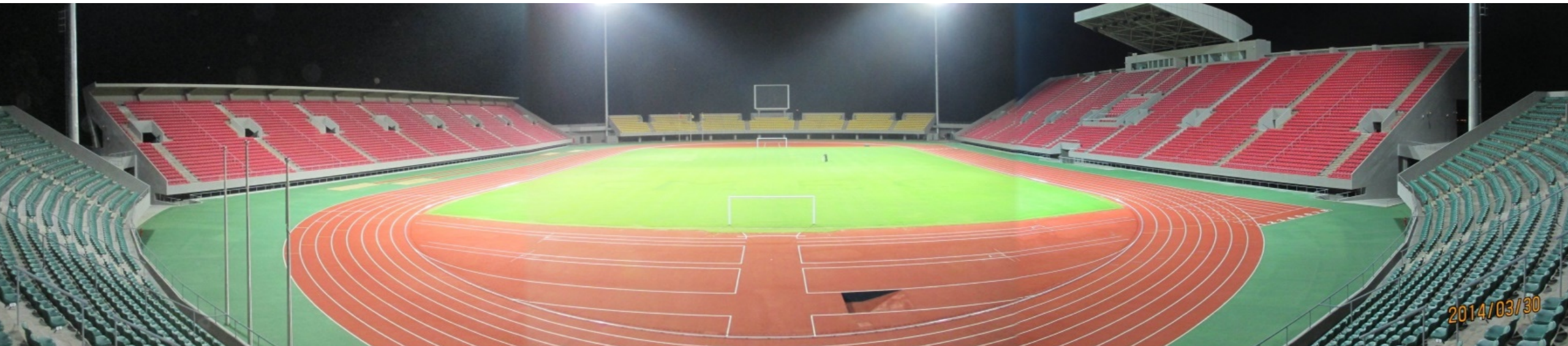
Limbe Stadium Project, Cameroon
