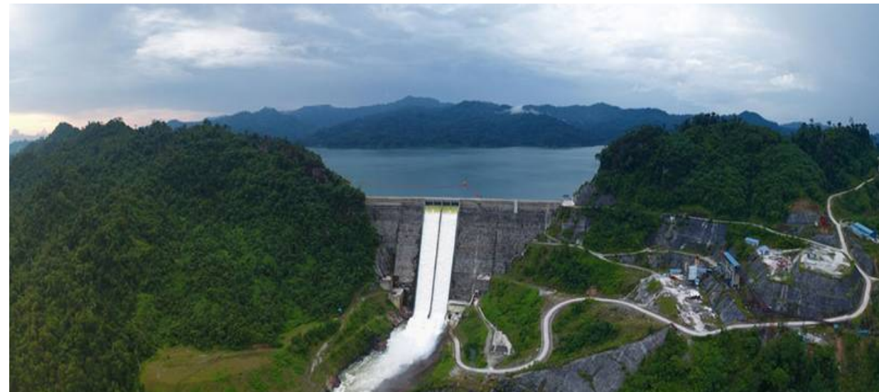
Murum Hydropower Plant ,Malaysia (4*225MW)
