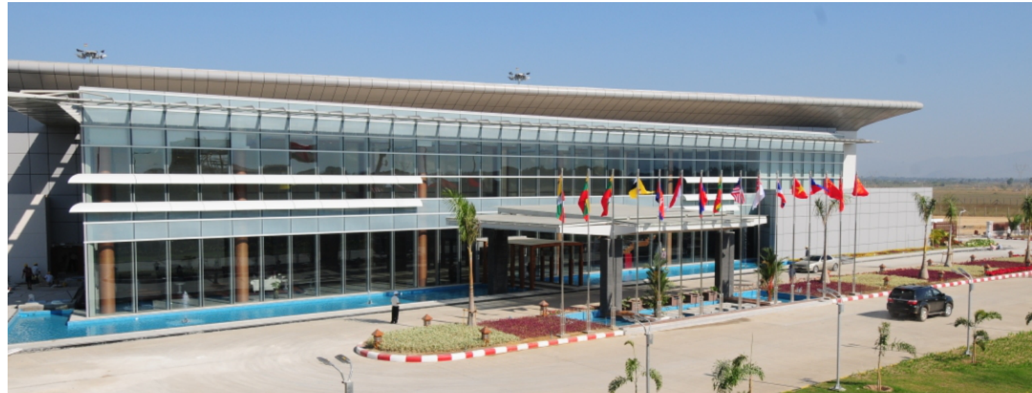
Nay Pyi Taw International Airport Project,Myanmar
