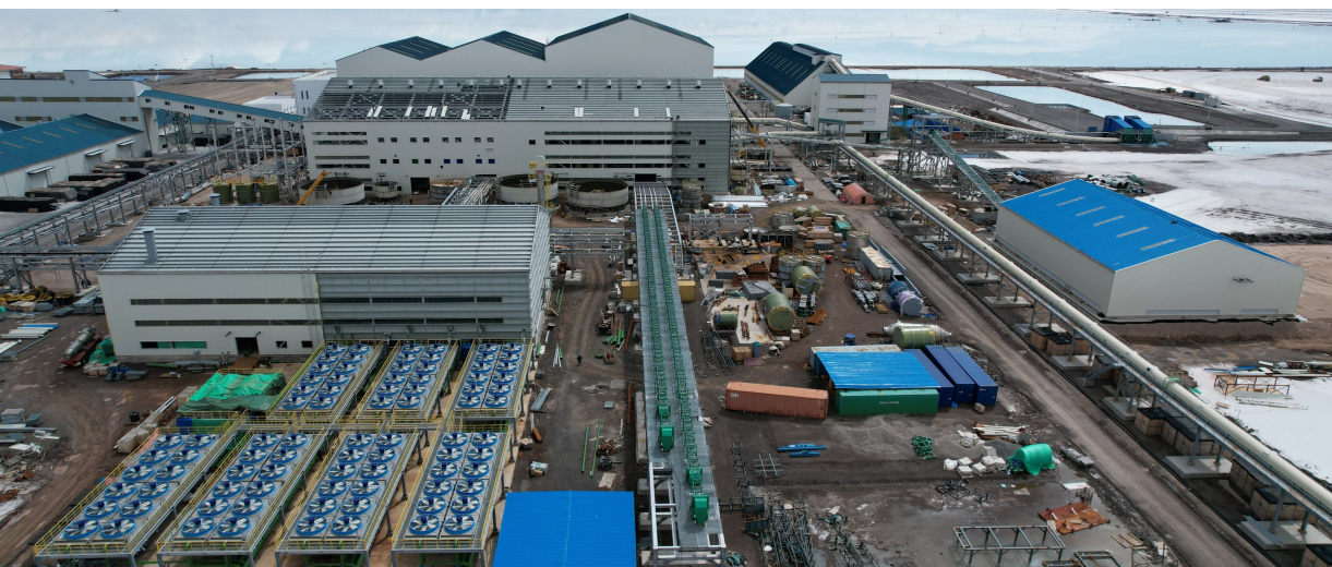
Construction, Assembly and Commission of the Lithium Carbonate Industrial Plant
