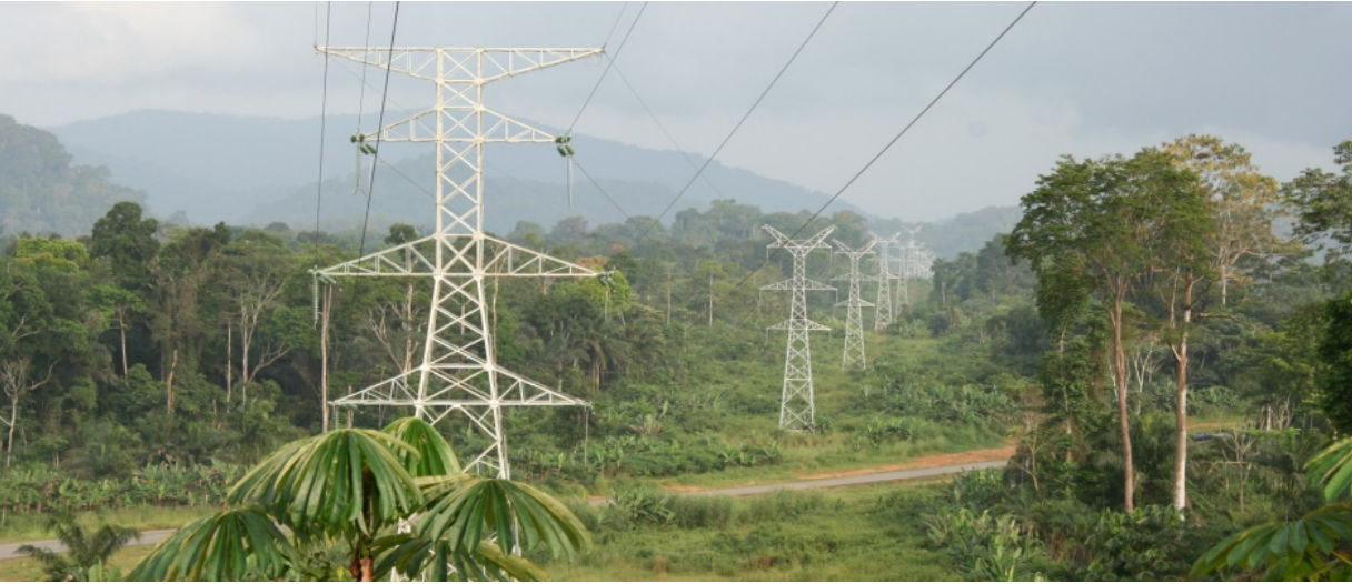
Transmission Line and Substations for Djibloho Hydropower Plant, Equatorial Guinea
