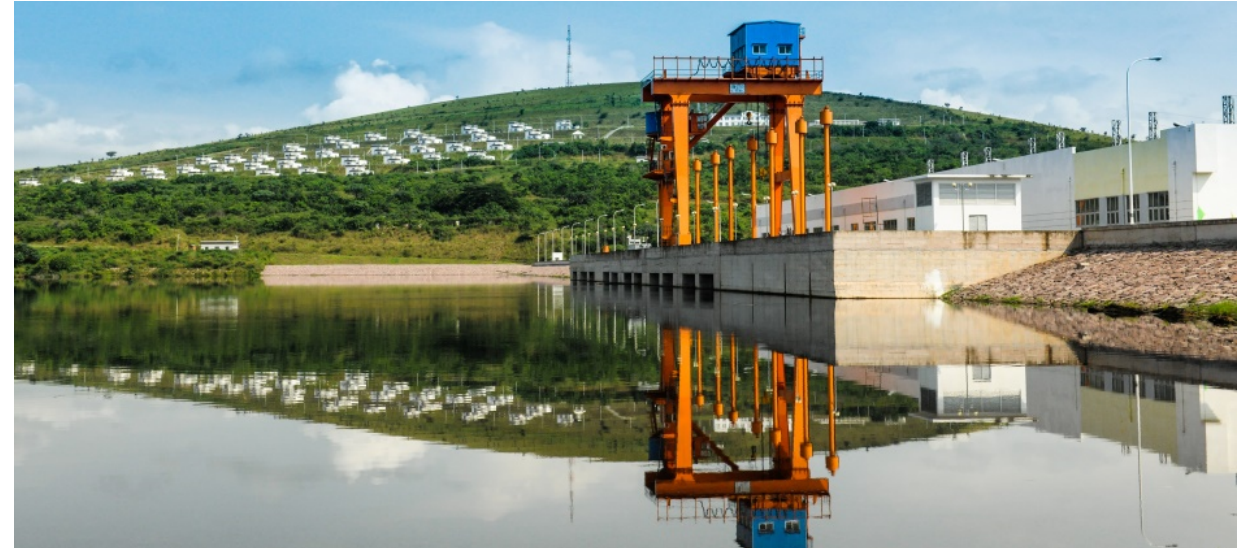
Imboulou Hydropower Plant ,Congo(Brazzaville) (4*30MW)
