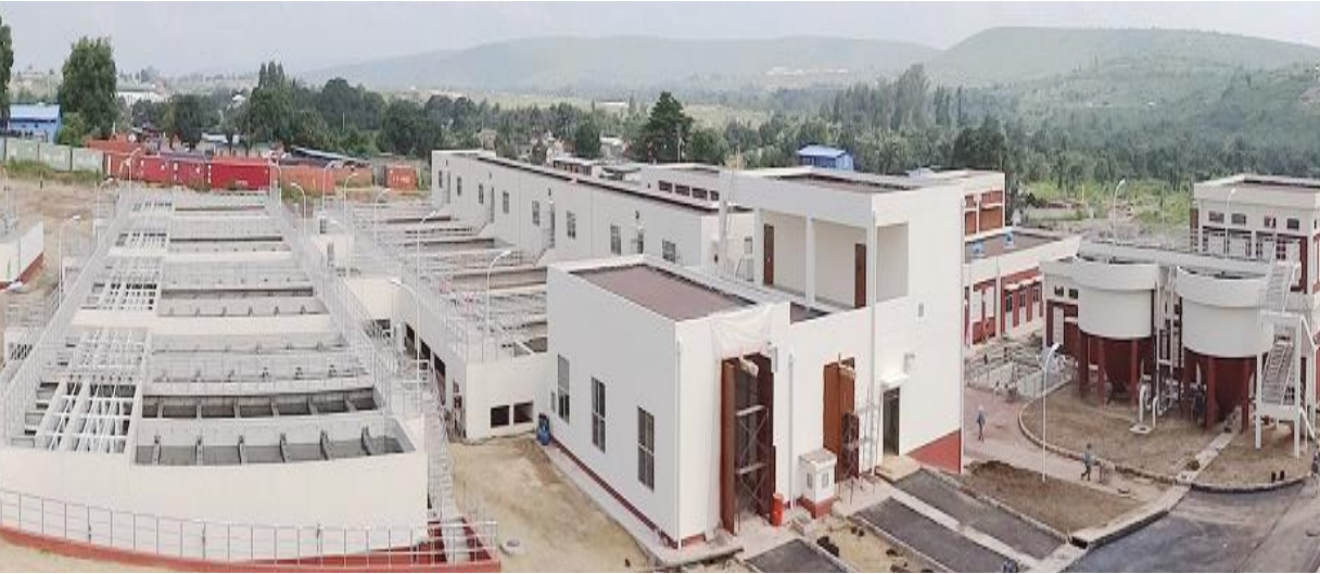
Djiri Drinking Water Treatment Plant Project, Congo(Brazzaville)
