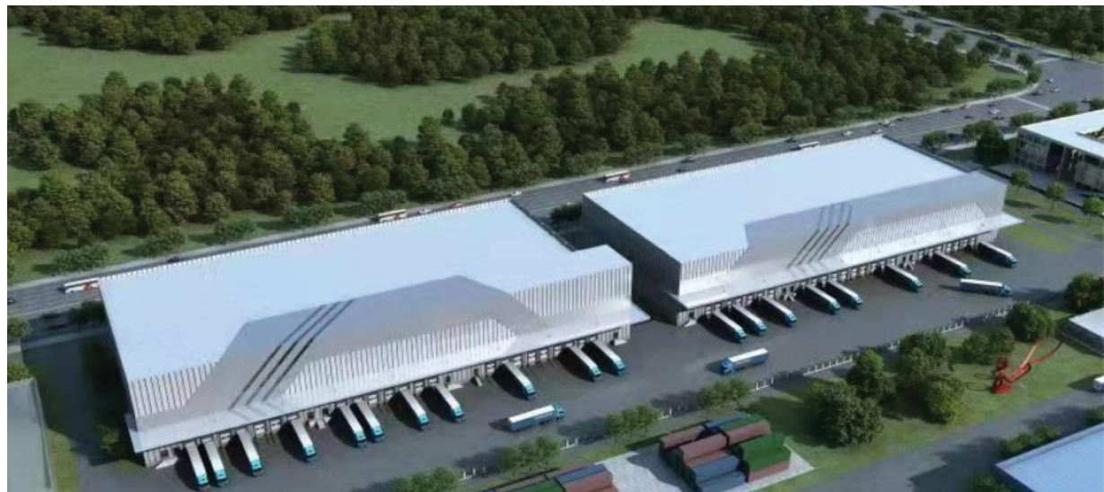
Beijing Qianxi Crane Cold Chain Logistics Project
