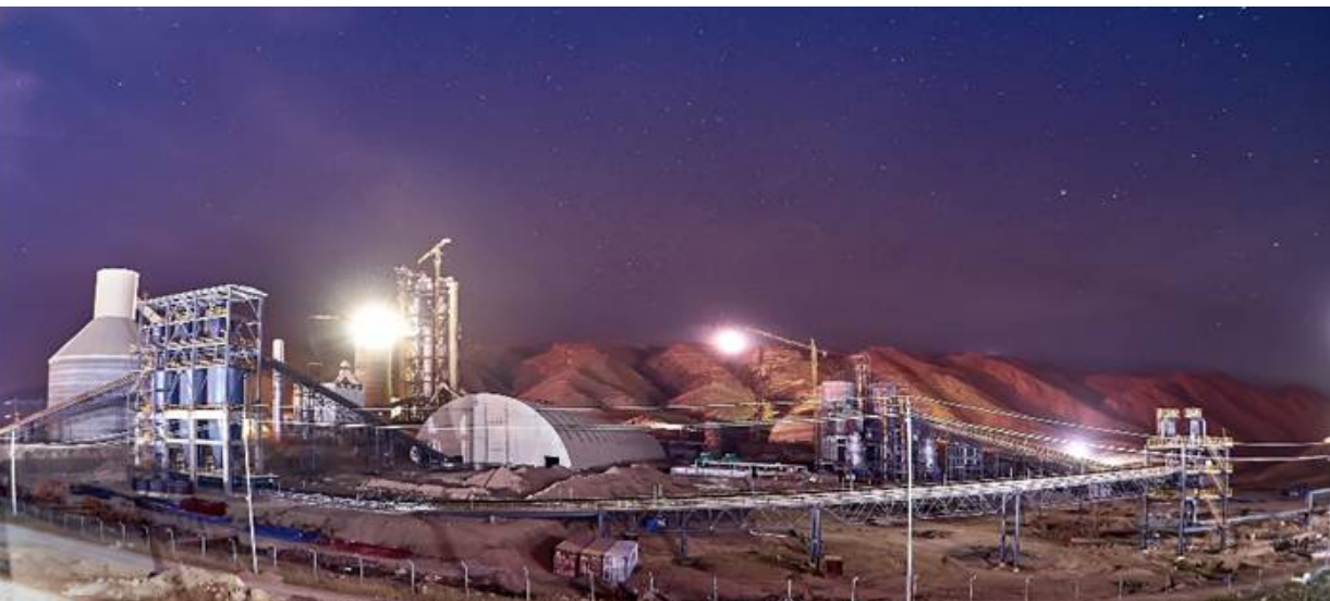
KAR Group Cement Plant in Qarachog,Iraq
