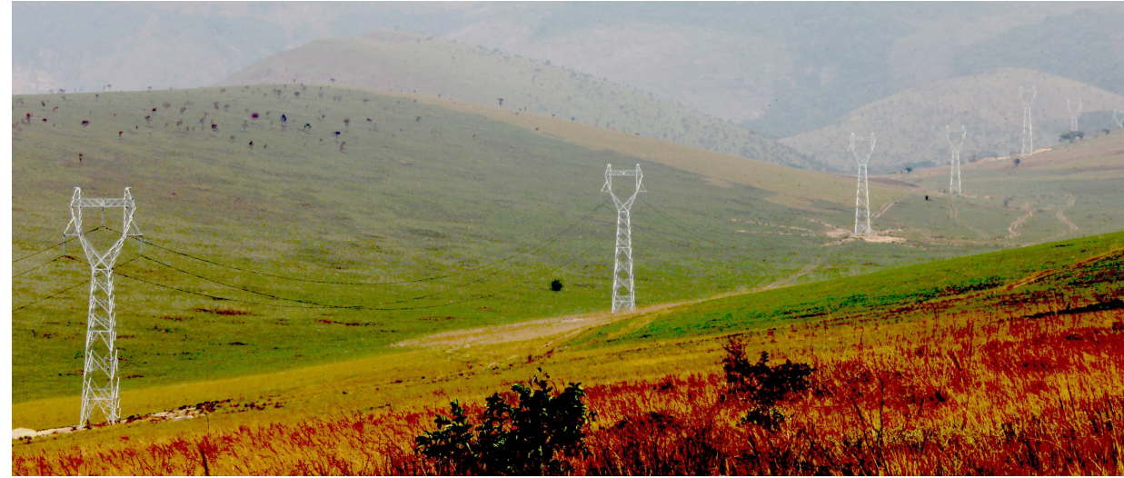
Transmissionline Project in Congo(Brazzaville)
