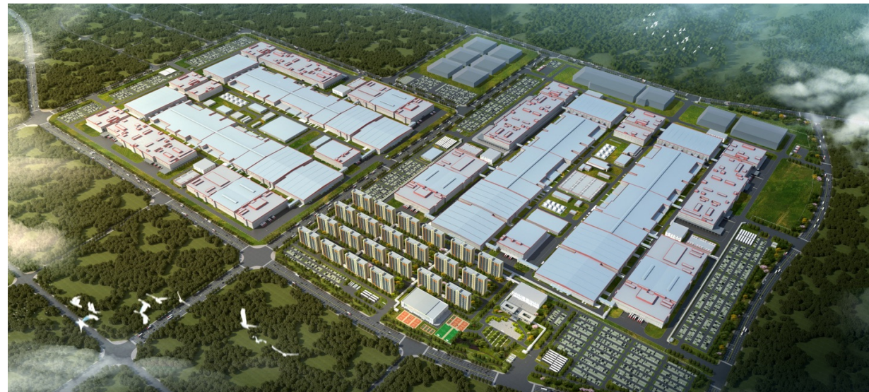
CATL Sichuan Power Battery Manufacturing Base P5 Project
