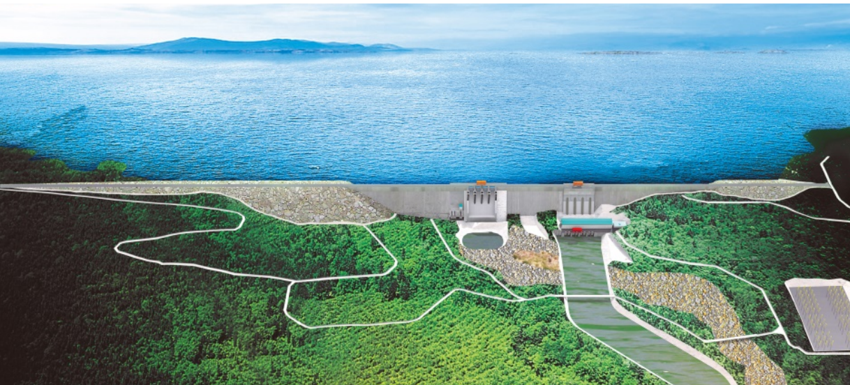
Zungeru Hydropower Project,Nigeria (700MW)
