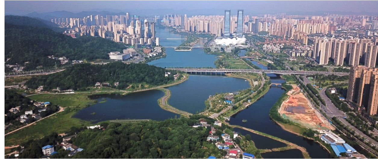
Smart Water Project (Phase I) of Longwang Port Basin in Xiangjiang New District, Hunan Province
