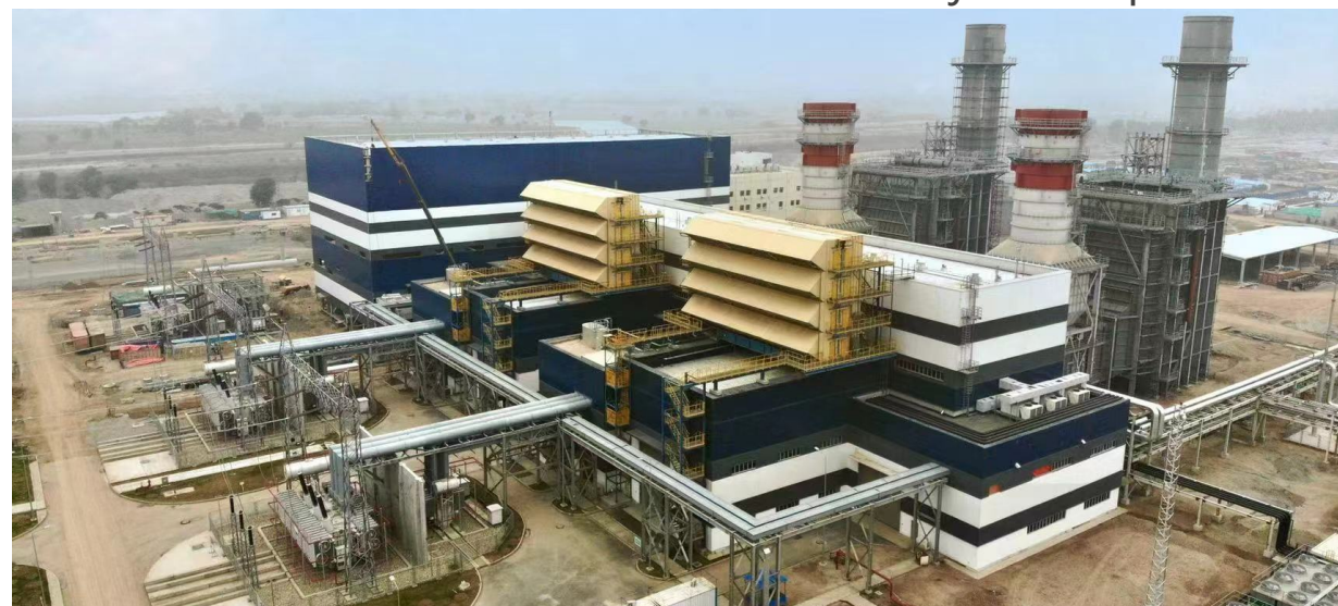
Jhang 1263MW Combine Cycle Power Plant Project, Pakistan
