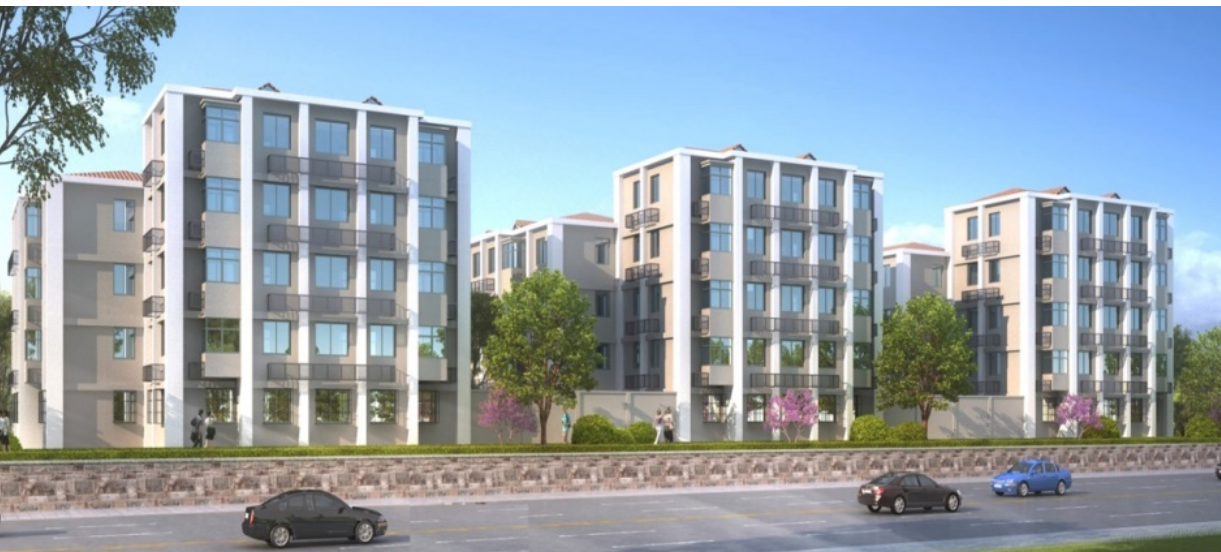
Renovation of Old Residential Communities in Beijing
