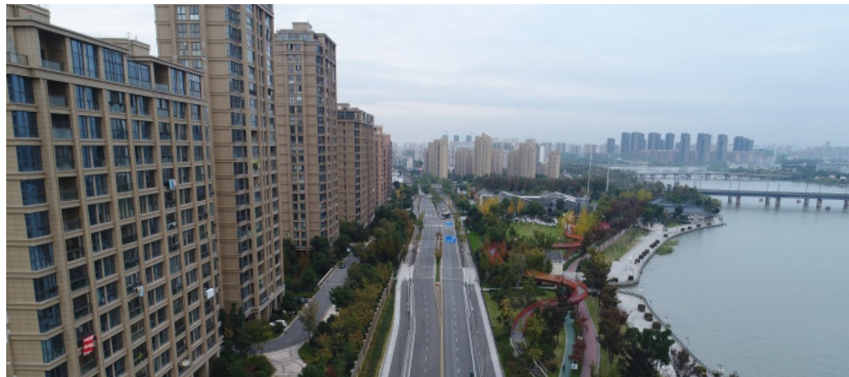
Sponge Renovation Project in Xiejia and Tianshui District of Ningbo City
