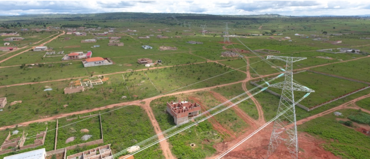
Lauca 400kV Transmission Line Project, Angola
