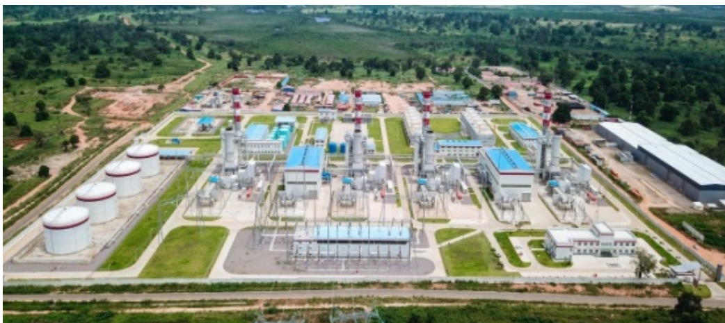
Soyo I Combined Cycle Power Plant
