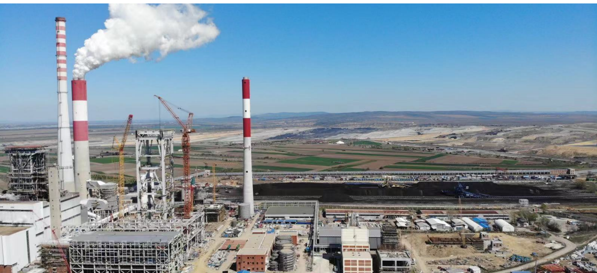
The Package Project of KOSTOLAC-B Power Plant, Serbia
