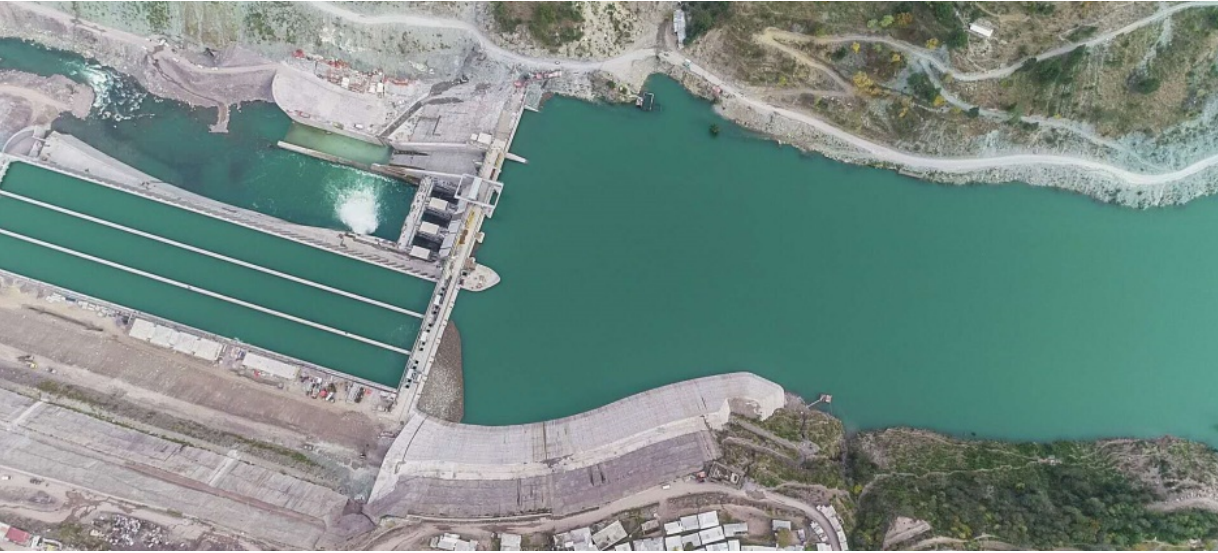
Neelum - Jhelum Hydro electric Project,Pakistan (4*243MW)
