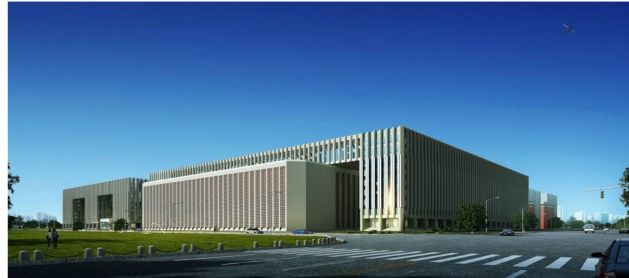
Tencent Internet Data Center Project
