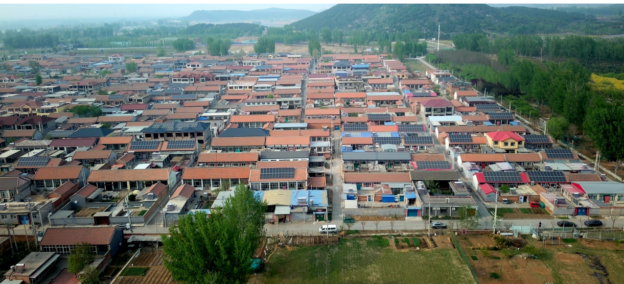
Beijing Shunyi District 26.88MW Household Distributed Photovoltaic Project
