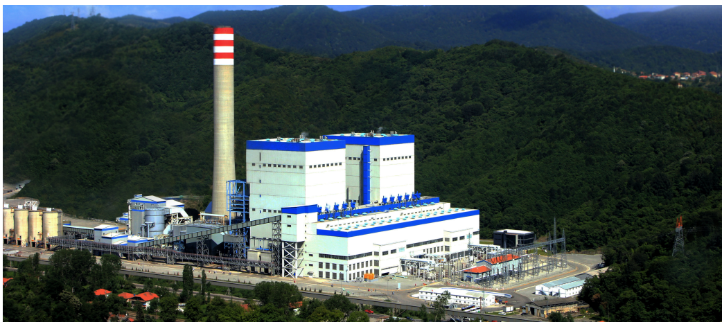
Eren (1+1) *600MW Supercritical Coal-fired Power Plant
