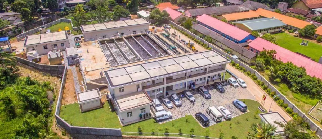
Kulunegala Sewage Treatment Plant , Sri Lanka
