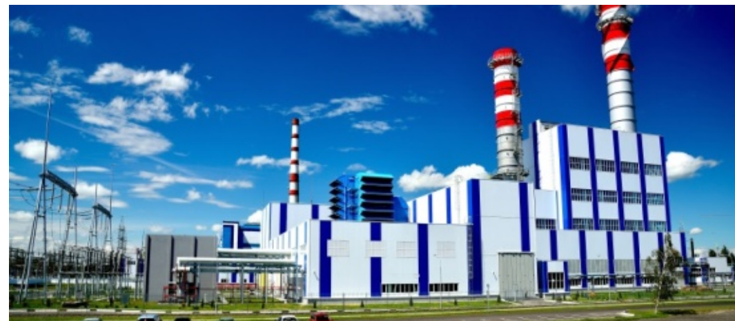
Berezovskaya 427 MW Combined Cycle Power Plant
