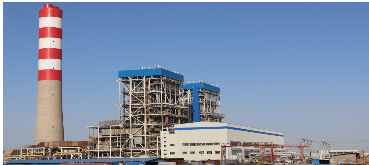
Salah Aldin 2x630MW Power Plant Project, Iraq
