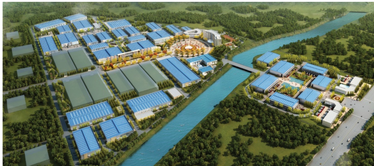
CRRC Yongji Intelligent Manufacturing Logistics Park
